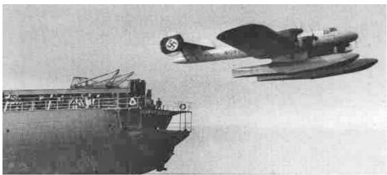
These "Wales" were mounted on steam catapults on the deck of the ship and could be started and refueled this way easily.
